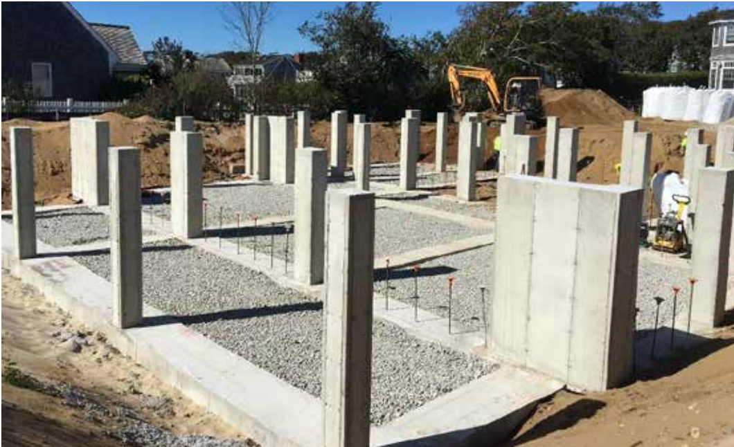
SUB-SLAB INSULATION & CAPILLARY BREAK
