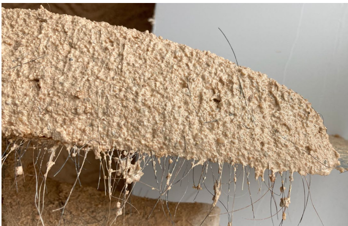
Image of properly haired base coat of plaster. Approx one hair every 1/8 of an inch.
